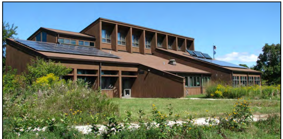
The system includes 66 solar panels (33 over the library and 33 over the auditorium) and two inverters. The raised solar panels visible on the far end are for our water heating system, which was installed during construction of the center in 1986.
